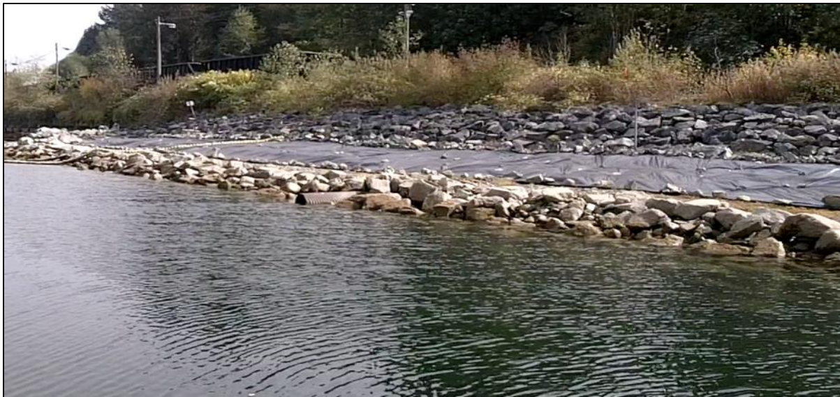
Figure 12. 2012 Pilot site of Geofabric control on S. patens in Burrard Inlet (Reed Point Marina)
